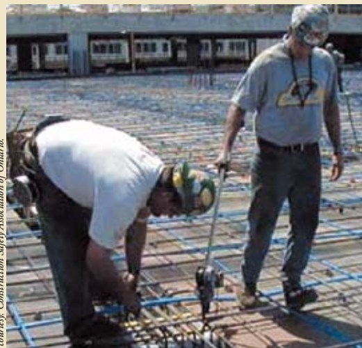
Manual rebar tying (left) vs. Use of an extended-handle rebar tying tool (right)
