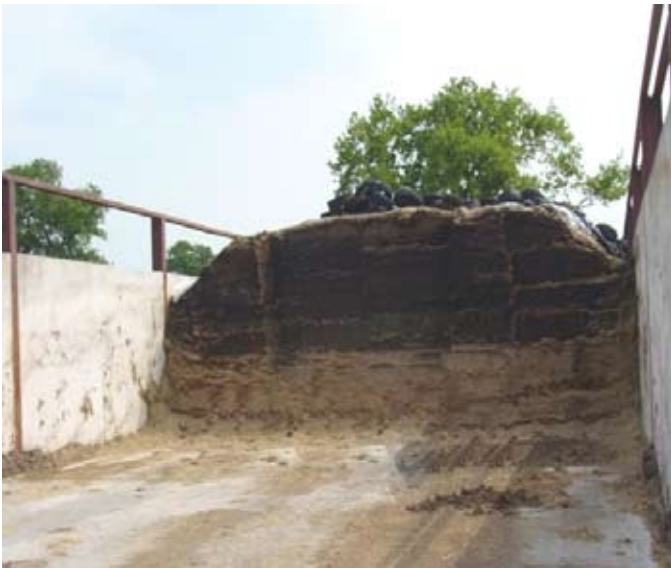
Figure 3. Sighting rails at the top of the bunker silo provide a visual clue while unloading silage.
