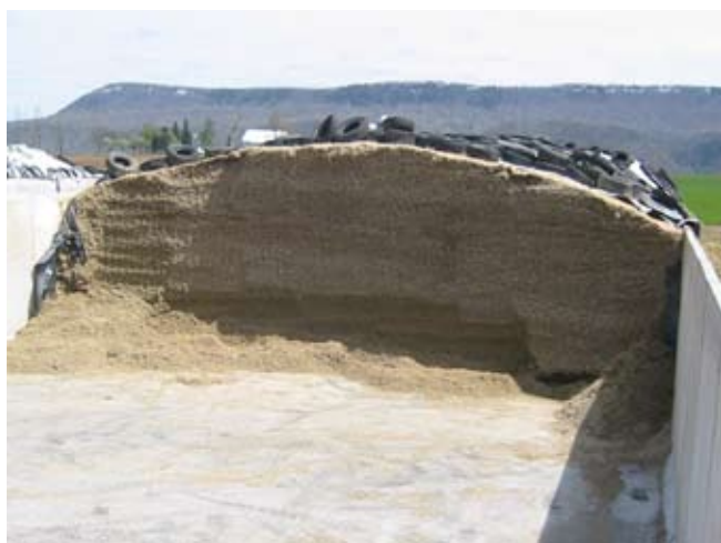
Figure 1. Bunker silos might have concrete or wooden post walls
