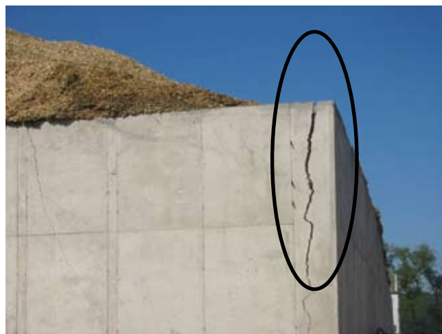
Figure 2. A cracked bunker sidewall needs repair.
