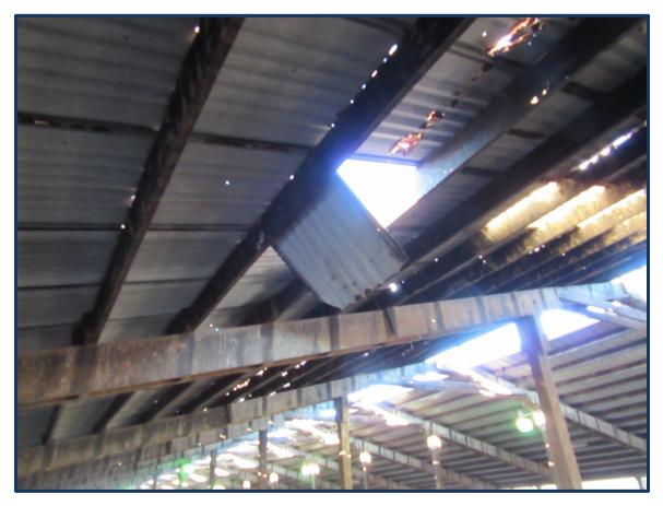
Incident scene showing part of the cow barn metal roof that gave way when the victim stepped on it and fell through, landing 12 feet below.
