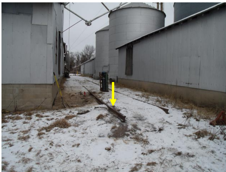
Figure 2. Identification (yellow arrow) and location of railroad spur being removed
