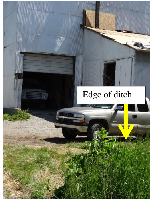
Figure 5. Embankment edge in relation to loading area.
