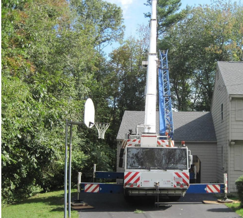
Figure 1 – Crane positioned in the driveway of the home
