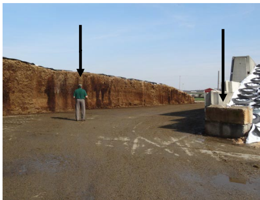
Figure 3. Bunker configuration change – note angle of cement compared to Figure 1 and approximate location of decedent.
