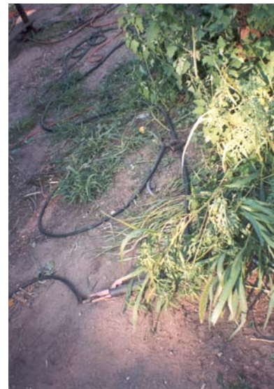
Figure 4. Un-insulated splice
