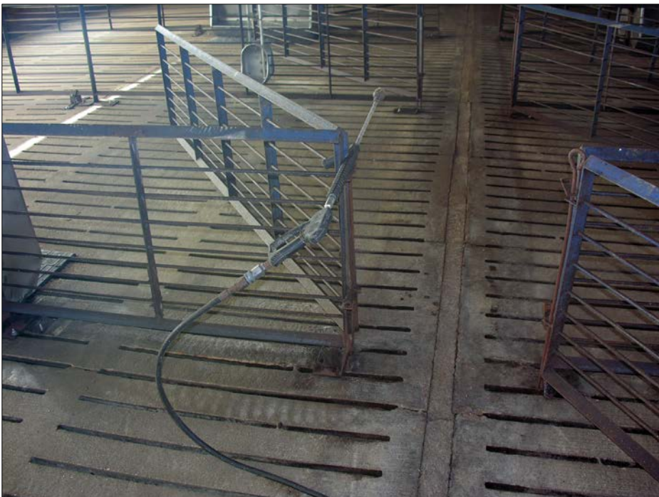
G. Scene inside the building (above and at left). Victim had been moved to loading dock area.
